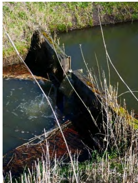
Foto 1.2. Stuw in watergang EVZ
